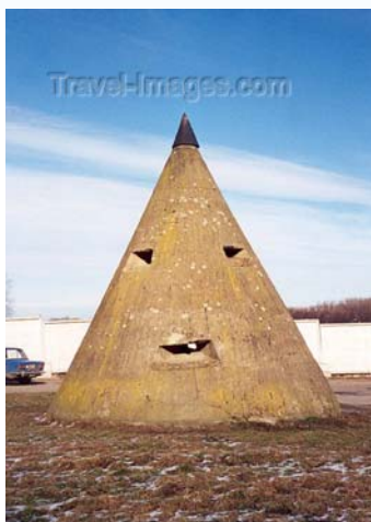
Be-145. Beton bunker
