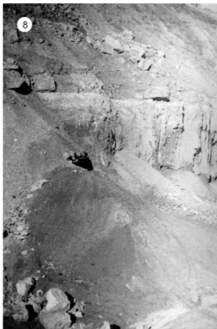
7. Dorottya I open pit (1958). Northern wall of the open pit. Lower part bauxite, upper part Middle Eocene limestone.
